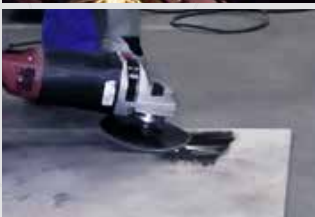
Removal of imperfections
