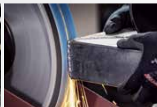
Levelling of welded seams
