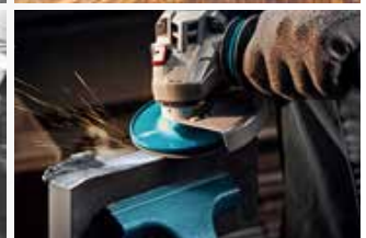
Removal of burn marks
